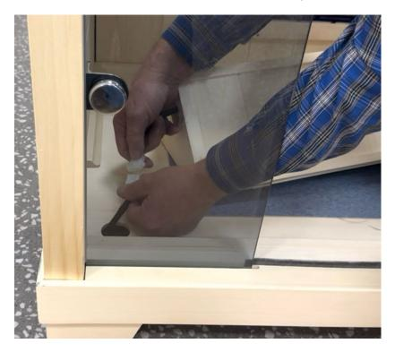
Push the excess cable into the floor so that it will not get in the way when the heater is installed.
