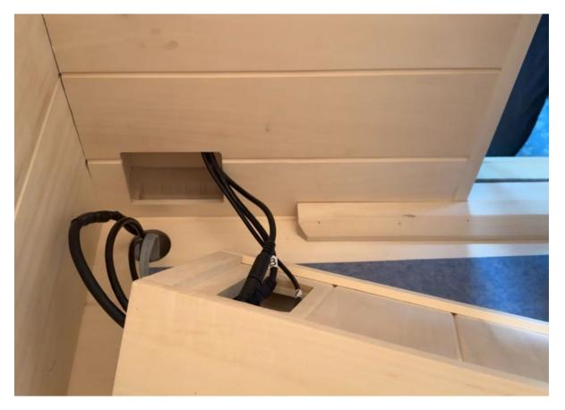
Notice the metal hook on the right side panel and the corresponding metal hook on the heater. Use these two hooks to secure the heater to the side panel the way you did with the left front heater. The easiest way to accomplish this is to align the heater against the side panel about an inch or two above its final position and then lower it into place:
