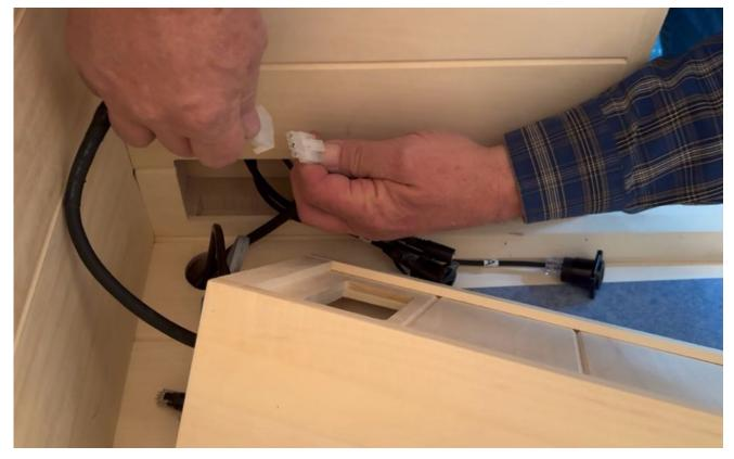
The remaining cables from the floor will pass through the floor side of the front heater out it's back side to connect with cables from the front panel.
