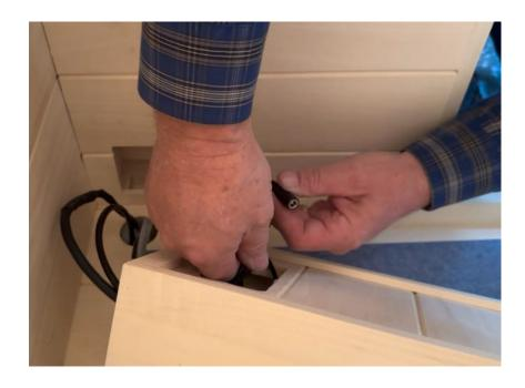
Tuck the connectors into the front heater or into the floor to get them out of the way. Tuck as much of the extra cable length into the floor panel as well. It should look something like this:
