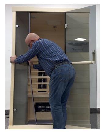
The other side of the magnet attaches to the side of the door. Make sure the magnet aims towards the inside of the sauna such that it will contact the magnet on the other side. Push the magnet onto the door starting at the top and making your way down.
