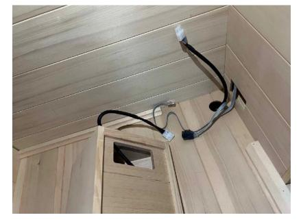
Pass the gray cable from the front panel through the side of the heater and out the bottom of the heater. Connect that cable to the gray cable from the floor panel.
