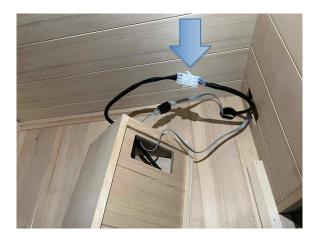
For front left heater (lift up heater to see connection):
