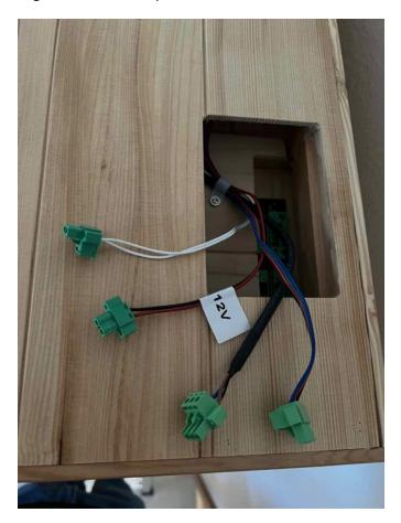
Two of the cables are the same size with 2 possible locations to connect them. The cable labeled "12V" will connect to the receptacle that is closest to the outside corner of the sauna.
