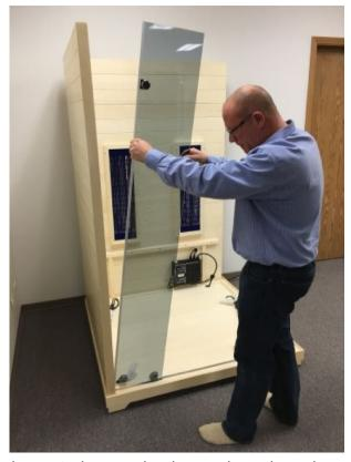
Note that if the glass is seated properly, the seal on the edge will sit evenly inside the groove in the left side panel.
