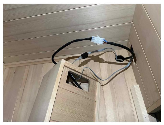
Tuck as much of the extra cable length with the connectors into the floor panel.
