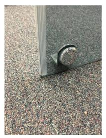
To place the side glass into the sauna, start by placing the bottom right corner of the glass in the floor panel. Then push the glass into the side panel:
