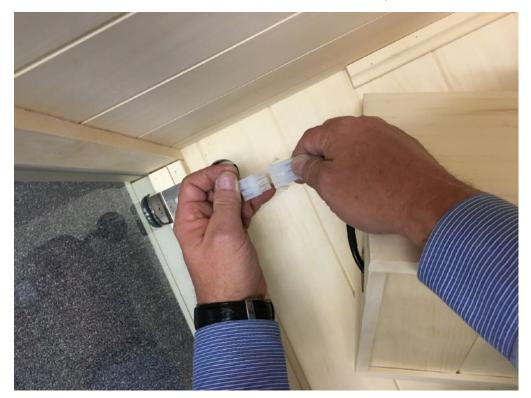
Push the excess cable into the floor so that it will not get in the way when the heater is installed.
