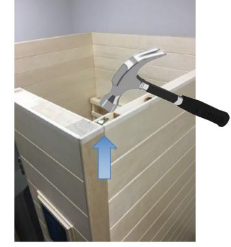
Add a screw to lock down the connection mechanism.
