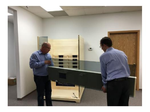
With the glass door still folded over the wood side of the front panel, place the bottom of the wood side of the front panel into the floor panel:
