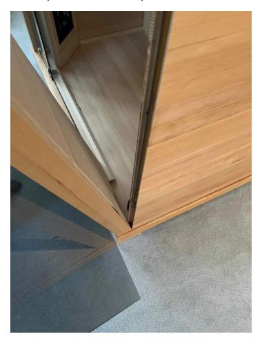
Before putting the front panel fully into place, make sure the right side panel's edge connection mechanism (located at the front of the top of the right side panel) is lifted up so that the "hooks" on the edge of the right side panel can insert into their matching slots on the front panel's edge. You can then complete the connection by tapping down the connection mechanism with a hammer -- have a second person hold the front wall panel while you do this to prevent the front panel from falling.
