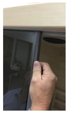
The other side of the magnet attaches to the side of the door. Make sure the magnet aims towards the inside of the sauna such that it will contact the magnet on the other side. Push the magnet onto the door starting at the top and making your way down.
